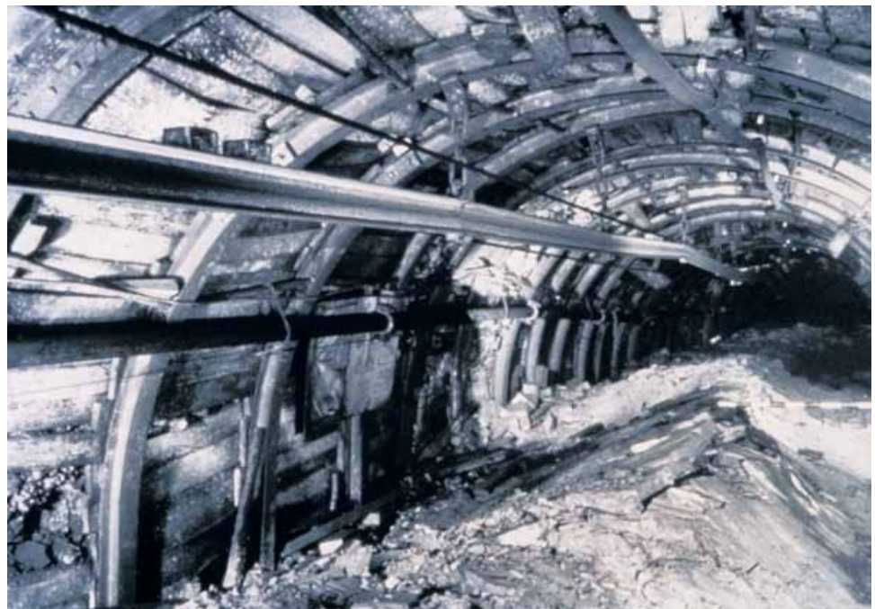
Figure 1 Looking at the condition of existing roadways is one way of collecting information. In this case, the arch supports are standing well, but lateral stress is causing floor heave
