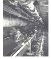
Figure 7 Conveyor manriding below ground
