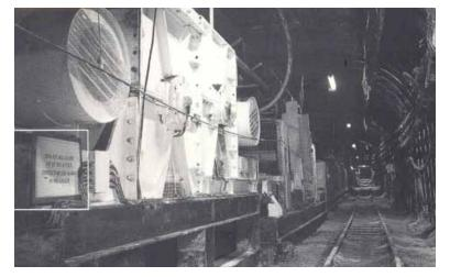
Figure 10 Notice giving location of isolating switchgear
