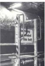
Figure 5 Integral lockable gate for use when manriding has been suspended
